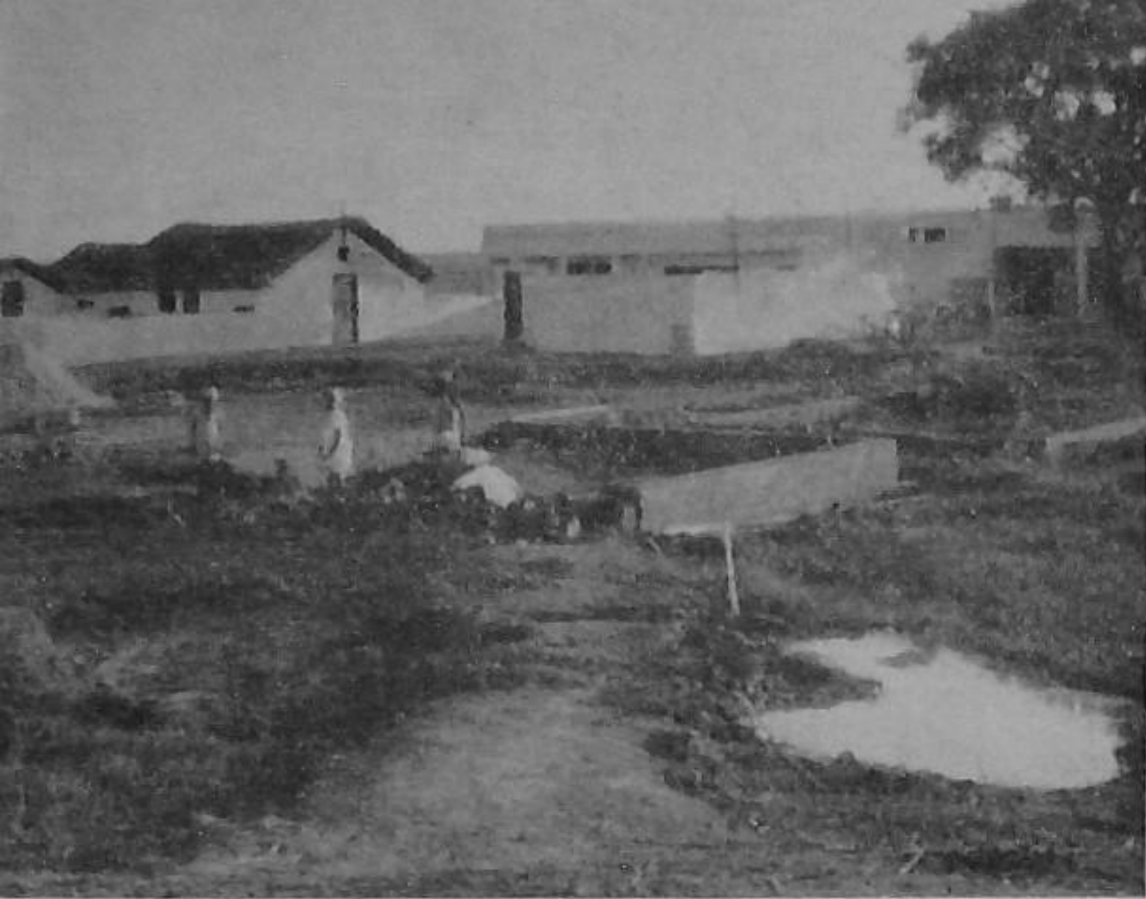
A view of the newly constructed sheds and buildings for poultry and piggery units set up by the Panchayat Samiti, Nilokheri
