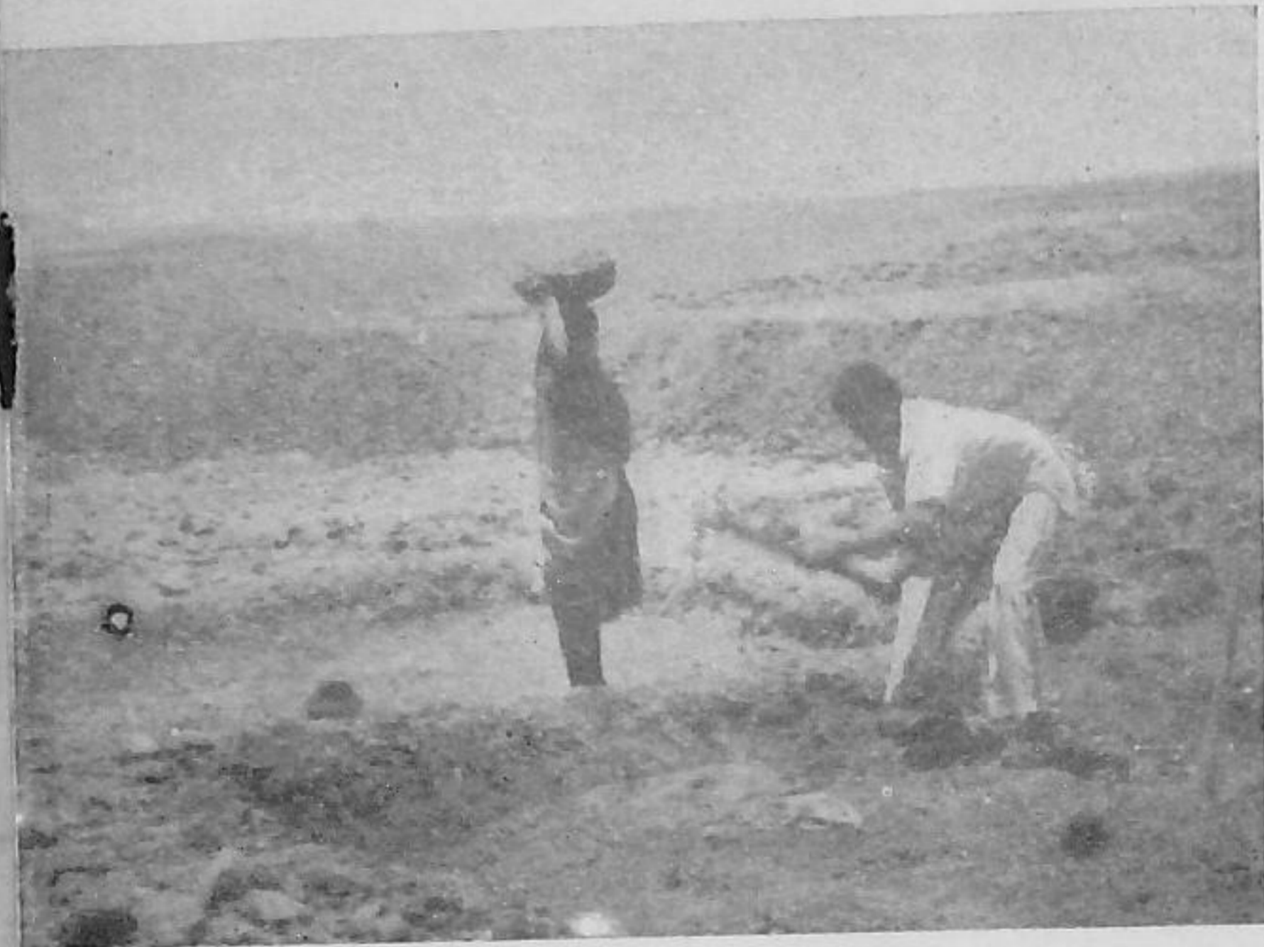
For conservation of moisture in dry and arid areas like this one, contour bunding offers an effective solution.
