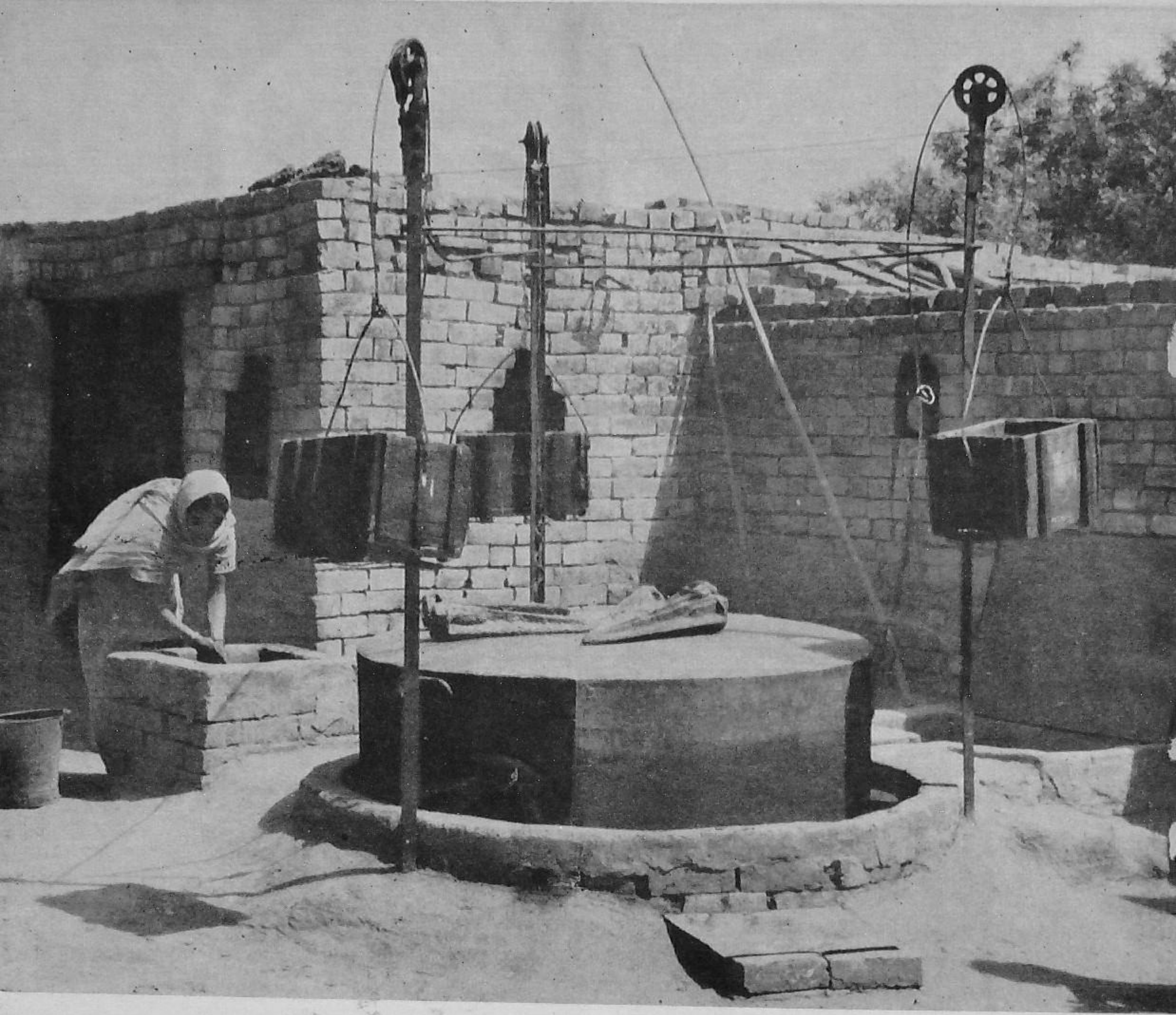
Cowdung Gas Plant in service for the last 6 years in Shri Laksi Ram's house in Nangloi village, Delhi State.
