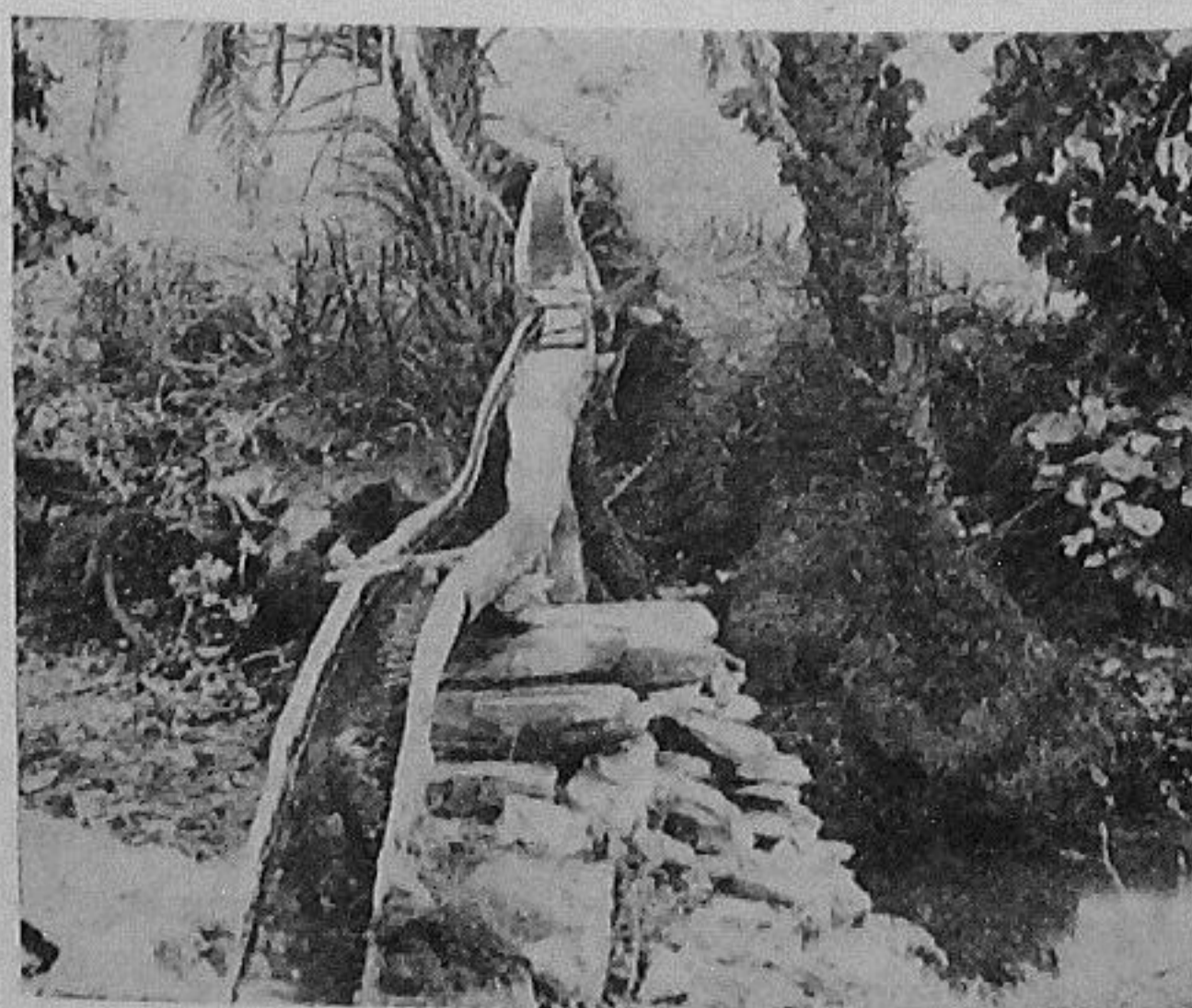
SARAN—a typical irrigation channel dug by the Adivasis by constructing earthen dams across hilly rivulets
