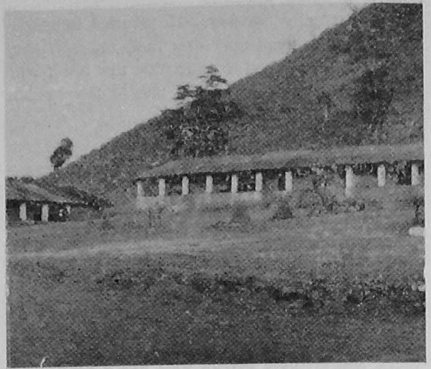
A view of a group of twelve houses and a Community Centre built at Limbada to encourage community living.
