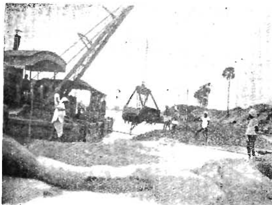
Dredger at work
