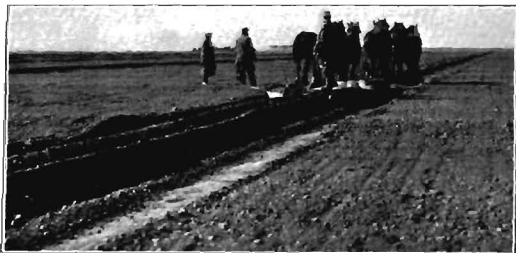
Fig. 6.—Grading Operations at Central Research Farm. Throwing up Banks with Check Banker.
