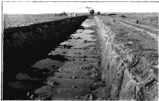
Fig. 3.—New Channel across Island Bend.
