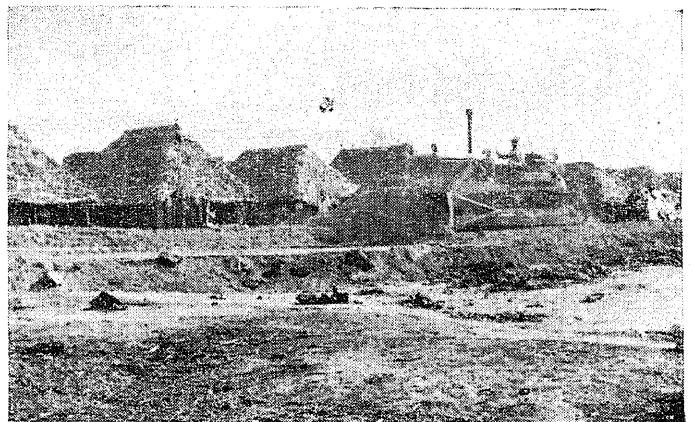
The Bulldozer at work.
