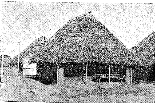
Dwellings under construction.
