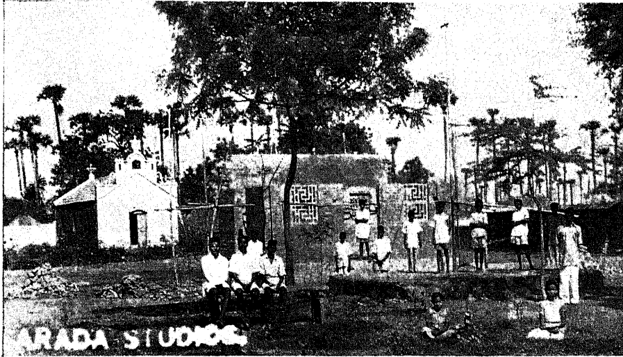
View showing the Building under construction as Mahatma's Memorial. It is intended for free library by the Panchayat Board, Mangalagiri. The boys are the inmates of Sri Kasturba Technical Institute and orphanage opened by Hon'ble Mr. K. Chandramouli. All the inmates are Harijans learning in the High School classes and other Handicrafts.
