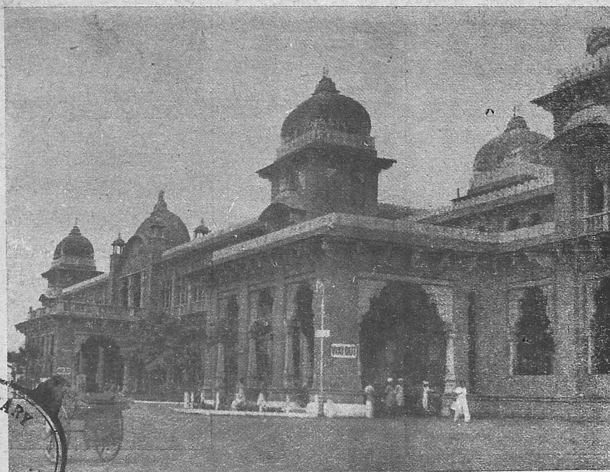
Egmore Railway Station
