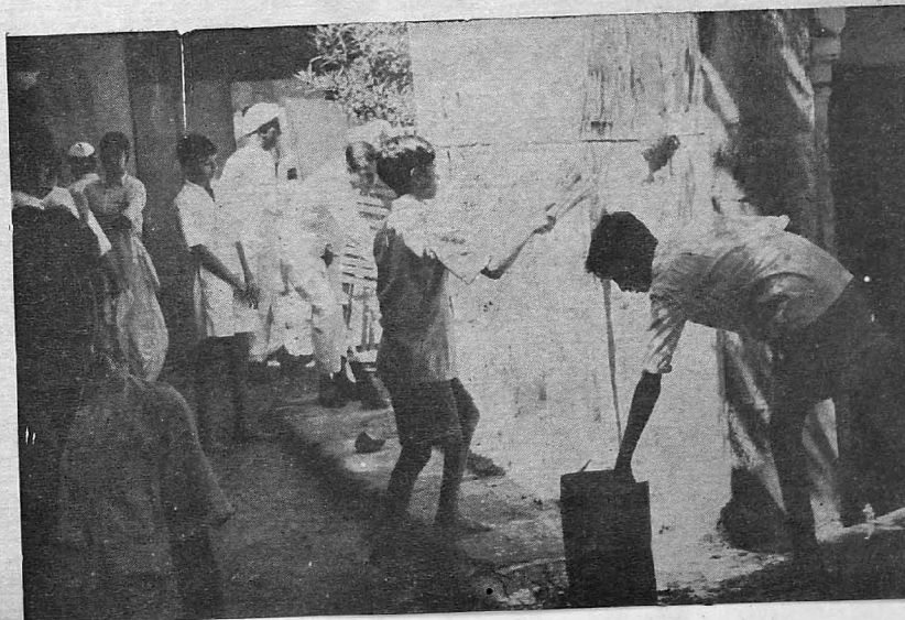
White-washing the temple walls.
