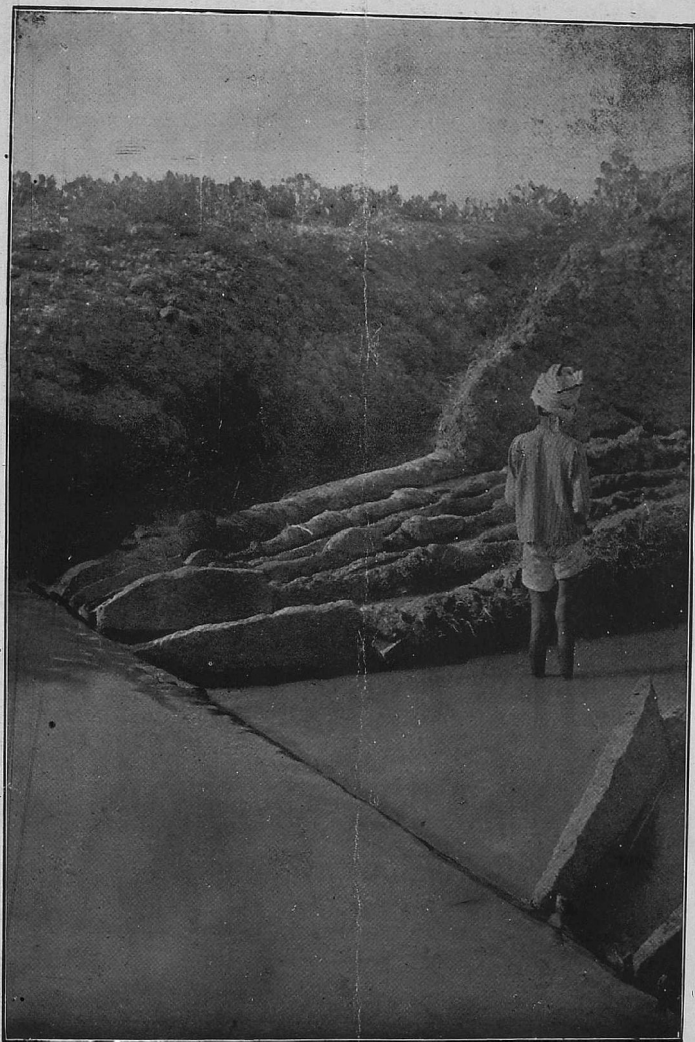
FIG. 3—Method of dividing water-supply (Chenganoor, Bellary district).
