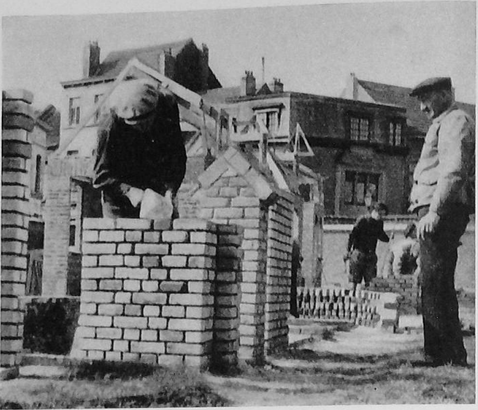
Centre for masons at Brussels, 1947. Bricklaying.
