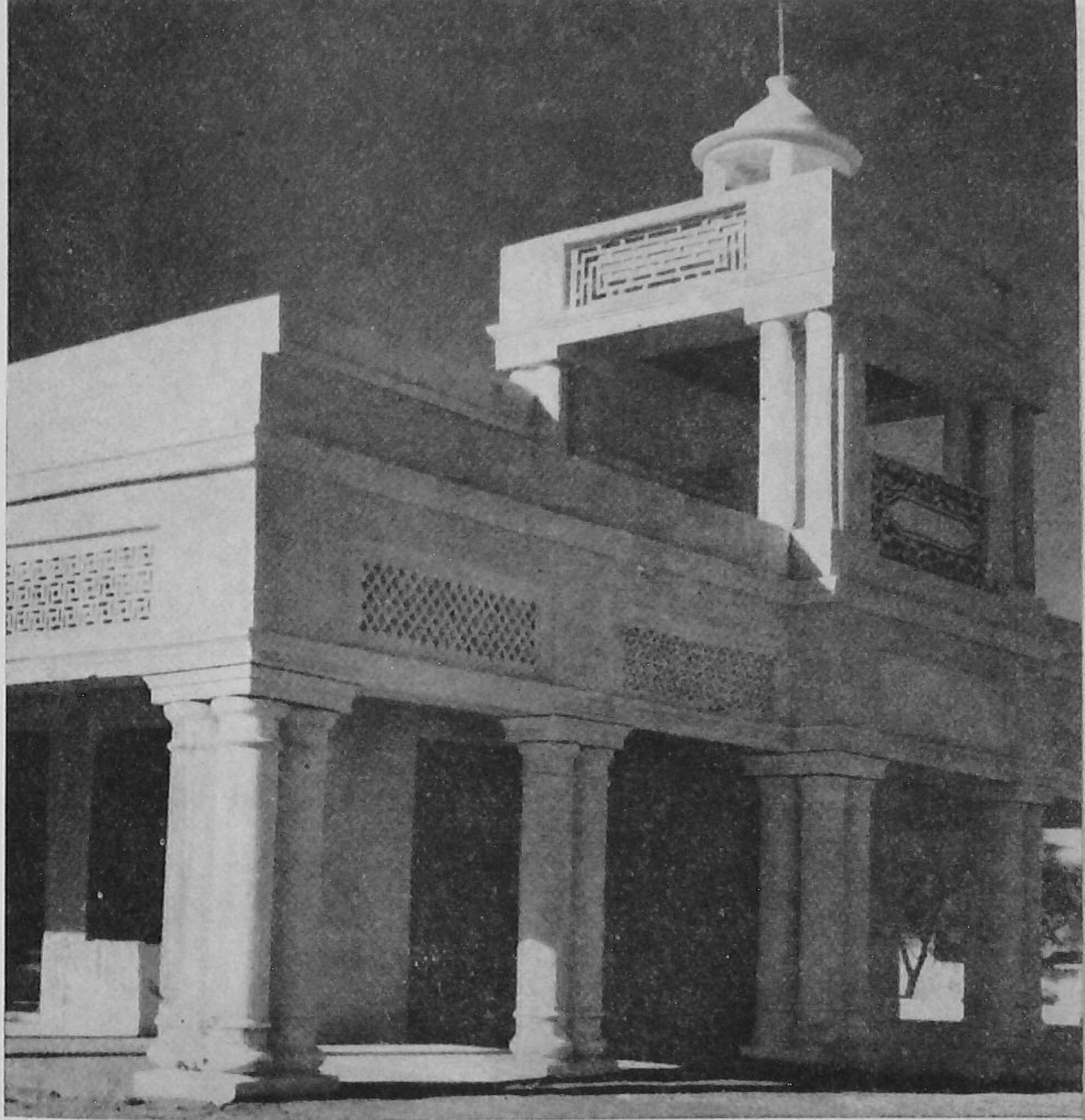
A view of the Community Centre in village Mukhmelpur
