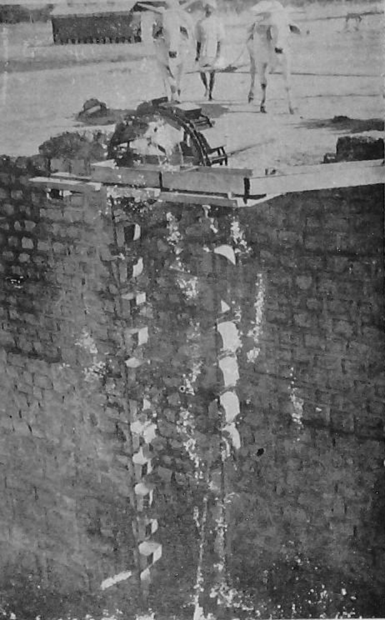
Persian wheel (showing chain of buckets inside the well)
