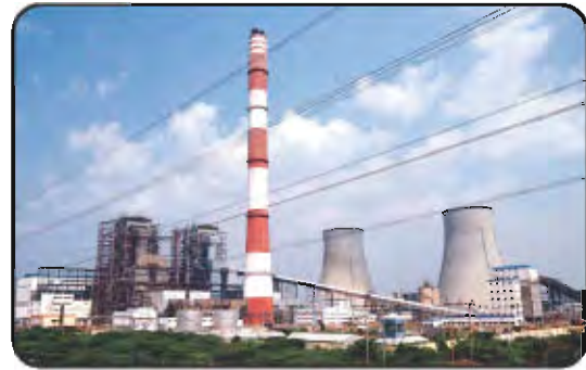
Thermal Power Station-Neyveli
