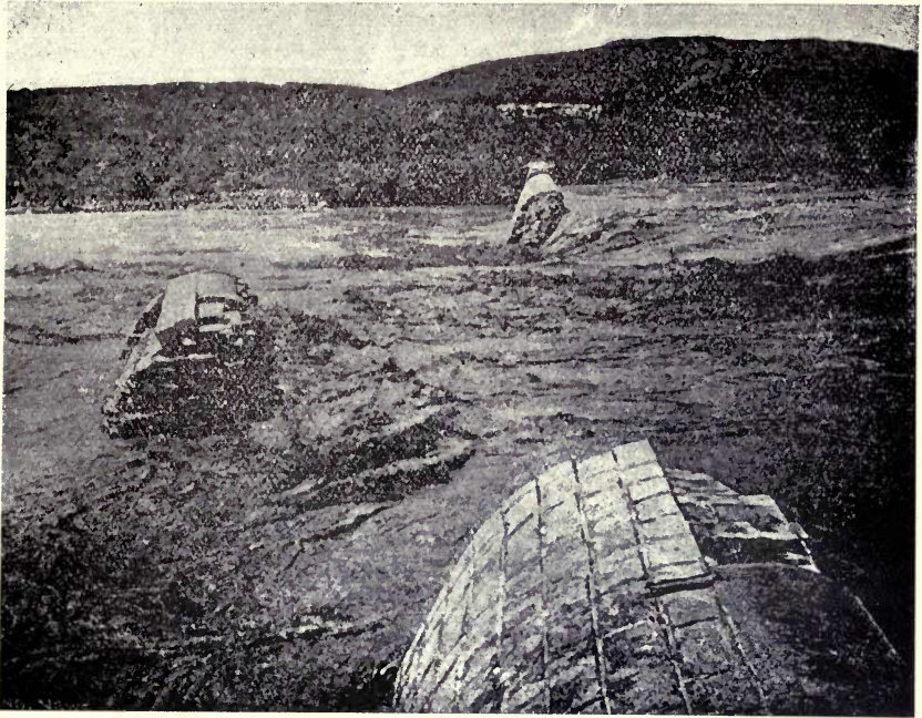
Plate II (a). Austin Dam, Texas. View taken during flood a few minutes after the break.
