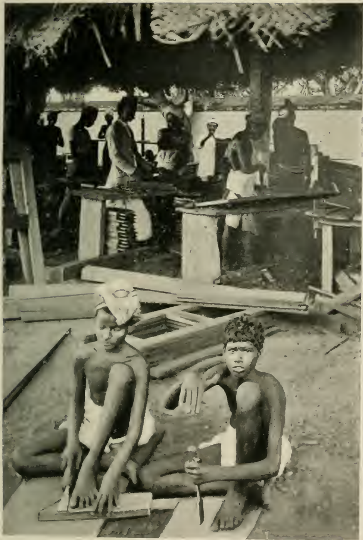
CARPENTERS AT WORK IN THE INDUSTRIAL SCHOOL AT TRICHINOPOLY. THE CHISEL IS STRUCK WITH THE PALM OF THE HAND.
