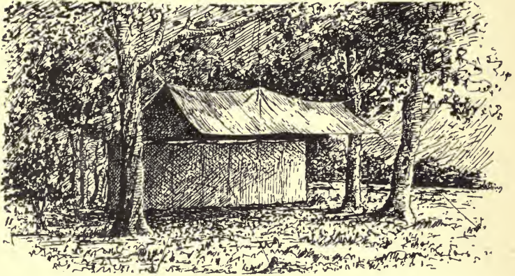
COOLIE SHELTER WITH WEATHER CLOTH ATTACHED
