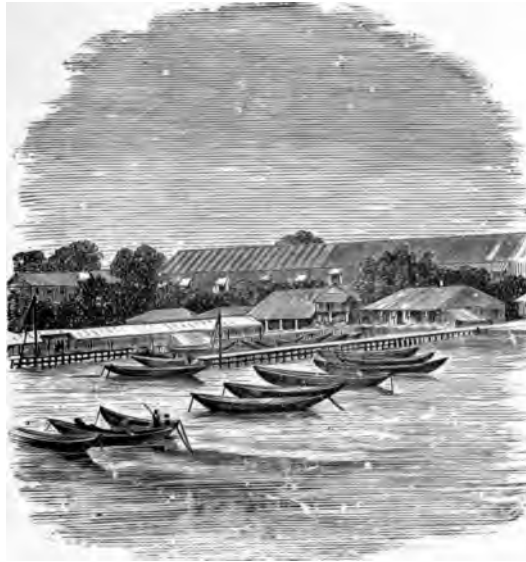
LANDING JETTY AT POINT-DE-GALLE
