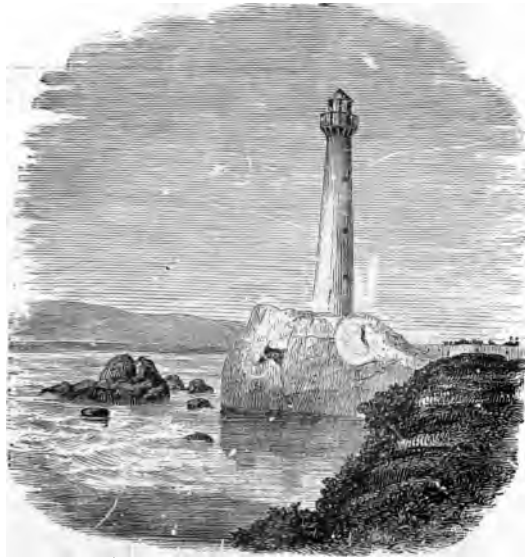
LIGHTHOUSE AT GALE.
