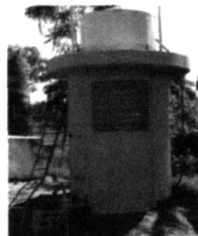
10 m 3 HIGH RATE REACTOR FOR CASSAVA STARCH FACTORY EFFLUENTS (SAGO EFFLUENTS)
