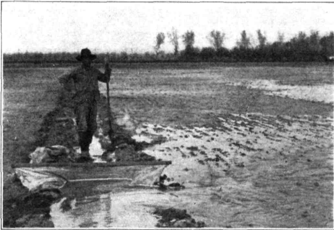
FIG. 38. Flooding with aid of canvas dam.
