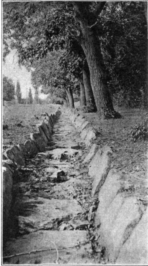
FIG. 19. Walled ditch to prevent erosion of easily "washed" soil.
