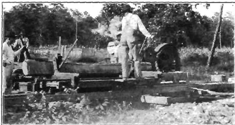
FIG. 268.—Saw mill showing dogs holding the log.
