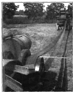
FIG. 184.—Tractor set about 18 inches out of line. This ruins a main drive-belt by stretching one side and wears it out by rubbing on the belt guide.
