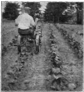
FIG. 295.—Cultivator with riding attachment.
