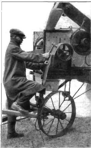
FIG. 309.—Covering a pulley.
