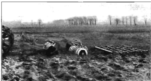
FIG. 65.—Disc harrow and peg-tooth used in combination.
