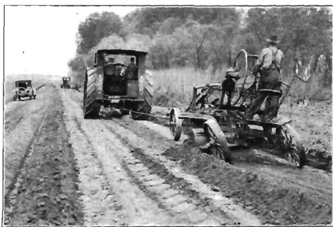
FIG. 170.—Heavy-duty road-grader and tractor. (Note lengthened hitch.)
