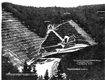
FIG. 139.—STEREOPHOTOGRAPHIC SURVEY FOR THE WISENTAL WATER POWER PROJECT SHOWING PERSPECTIVE CONTOURS, FOREBAY, PENSTOCKS AND POWER STATION.
