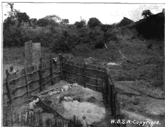
FIG. 106.—WELL-PROTECTED "SPRING" WATER SUPPLY AT SUMMIT. EAST AFRICA. SHOWING HOSE LEADING TO WATER-TANK
