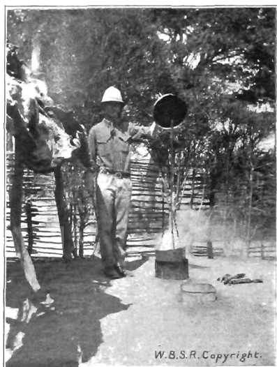
FIG. 99.—SMOKE URINAL, No. 1 CARRIER HOSPITAL, IRINGA SHOWING METHOD OF LOWERING BRAZIER
