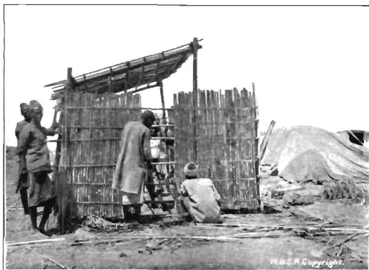
FIG. 78. LATRINE FOR DYSENTERY CASES, IN PROCESS OF CONSTRUCTION PORT AMELIA
