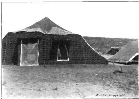
FIG. 127.—EXTERIOR OF FENESTRATED MUD-BRICK MOSQUITO- AND FLY-PROTECTED WARD, OF NO. 130 COMBINED FIELD AMBULANCE ON THE ROAD NORTH OF JAFFA Designed by Lieut.-Colonel OTWAY, R.A.M.C.
