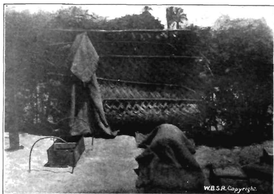
FIG. 83.—METHOD OF PROTECTING PAN CONTENTS IN INDIAN LATRINE FROM FLIES, AS SHOWN AT SANITARY DEMONSTRATION CENTRE DAR-ES-SALAAM
