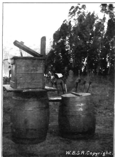
FIG. 91.—IMPROVISED LUMSDEN WET PRIVY OR HOME SEPTIC-TANK METHOD FOR DEALING WITH EXCRETA. Note fly-proof seat, closet barrel and effluent barrel. There is an anti-splash arrangement inside the closet barrel. Sanitary Demonstration Centre, Potchefstroom. Urine funnels seen in background.
