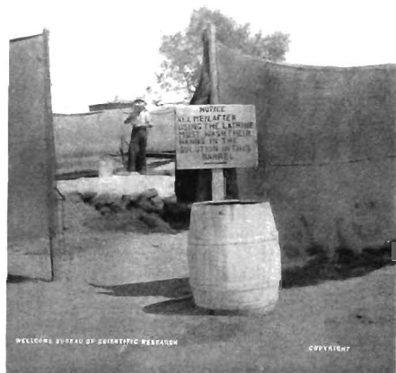
FIG. 114.—BARREL OF DISINFECTANT SOLUTION OUTSIDE A LATRINE
