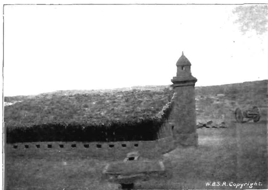
FIG. 100.—FENESTRATED MUD-BRICK COOK-HOUSE OF NO. 130 COMBINED FIELD AMBULANCE, ON THE ROAD NORTH OF JAFFA
