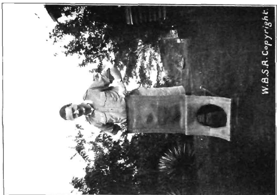
FIG. 81.-ADAPTATION BY THE GERMAN OF CAMP-STOOL FOR USE AS LATRINE SEAT
