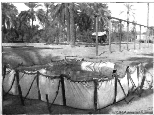
FIG. 107.—RUBBER CANVAS FOR HOLDING DRINKING-WATER. THESE CANVAS TANKS HOLD 2300 GALLONS
