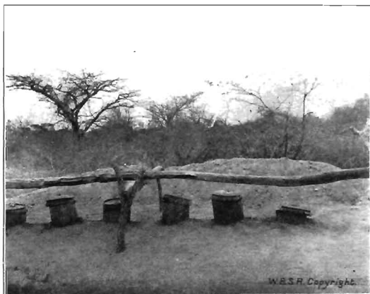
FIG. 92.—BAD TYPE OF TRENCH LATRINE, DODOMA The seat is uncomfortable and too high, there is no roof, and the covers of the cylinders leading to the pit are defective.
