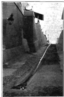
FIG. 22.—STREET SCENE IN CIUDAD BOLIVAR Showing central channel with stop-works and blocked grating.
