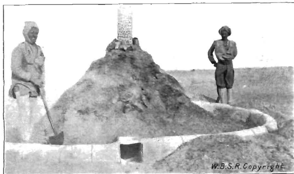
FIG. 87.—OPEN CONE INCINERATOR BEING USED FOR THE BURNING OF MANURE. Photographs 86 and 87 by CAPTAIN P. F. GOW, D.S.O., I.M.E.
