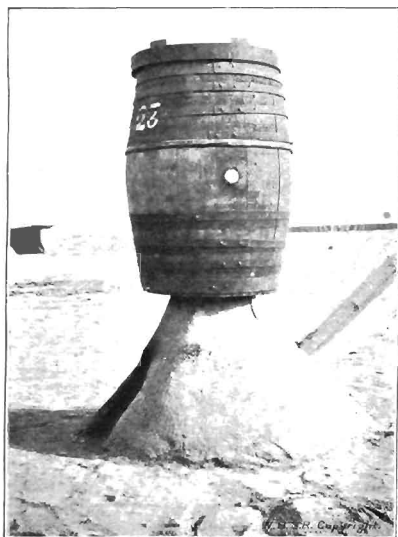
FIG. 120.—SERBIAN BARREL WRONGLY PLACED, MAKING IT DIFFICULT TO INSERT KIT IN THE BARREL OWING TO HEIGHT ABOVE GROUND LEVEL.
