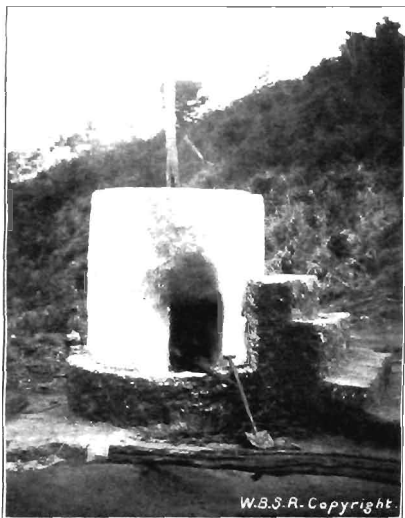
FIG. 88.—INCINERATOR PLACED ON CEMENT BASE TO PREVENT FLY-BREEDING.
