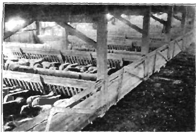
FIG. 152.—SHEEP BARN: INTERIOR VIEW, SHOWING ARRANGEMENT OF FEED-RACK AND METHOD OF DIVIDING THE PENS.
