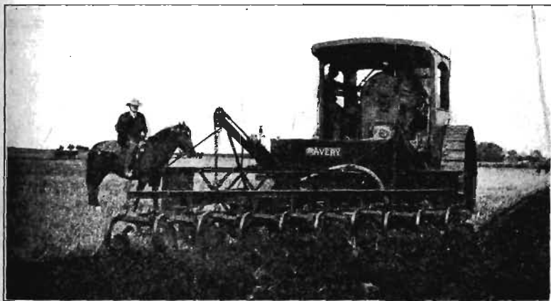
FIG. 41.—Gang plow, drawn by traction engine. Used for farming large areas.
