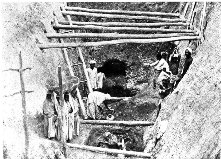
MICA : Making mine entrance safe, Jorasimar, Kodarma, Bihar and Orissa.
