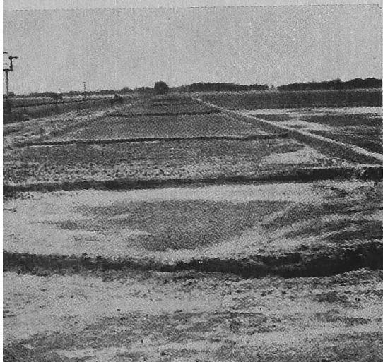
Compartment bunding for conservation of rain water
