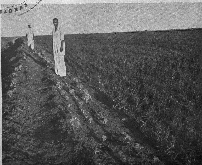
FIG. 2—Bunding : Area banded by bulldozers
