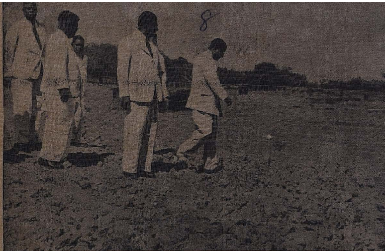
The Hon'ble Minister for Rural Welfare inspecting a site for a Harijan colony in Tanjore District
