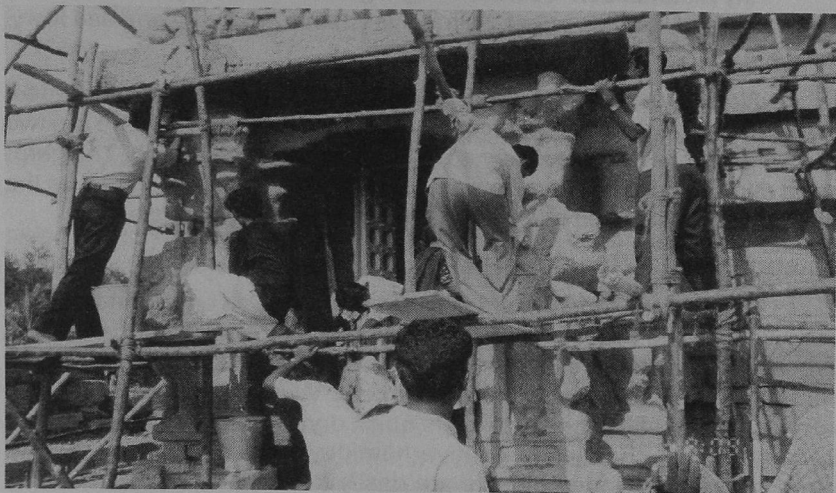
Removal of Salt by Poulticing at Shore Temple
