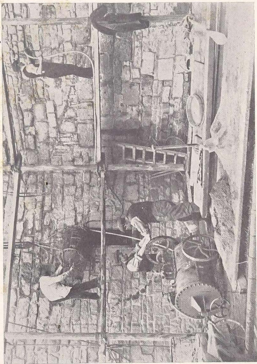
GROUTING MACHINE AT WORK (SEE PARA. 147).
