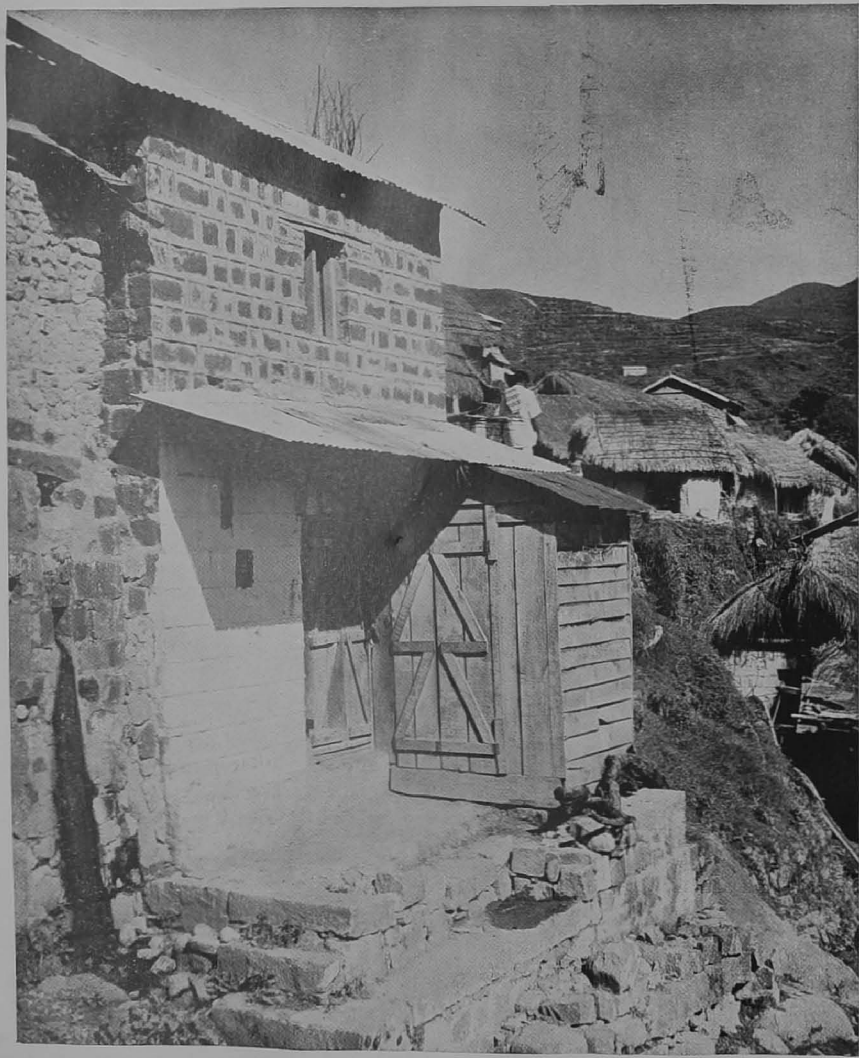
The Facade of a Vilpatti house. The uncared-for drainage - the uneven entrance the crude doors, and tin-sheet roofing.
