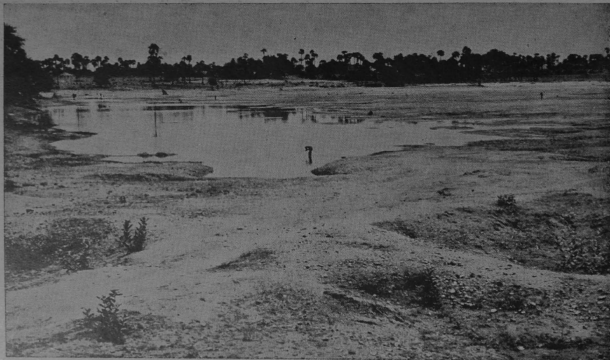
The source of supply to this tank is rain water. The scanty supply is barely sufficient to irrigate about 23 acres.
