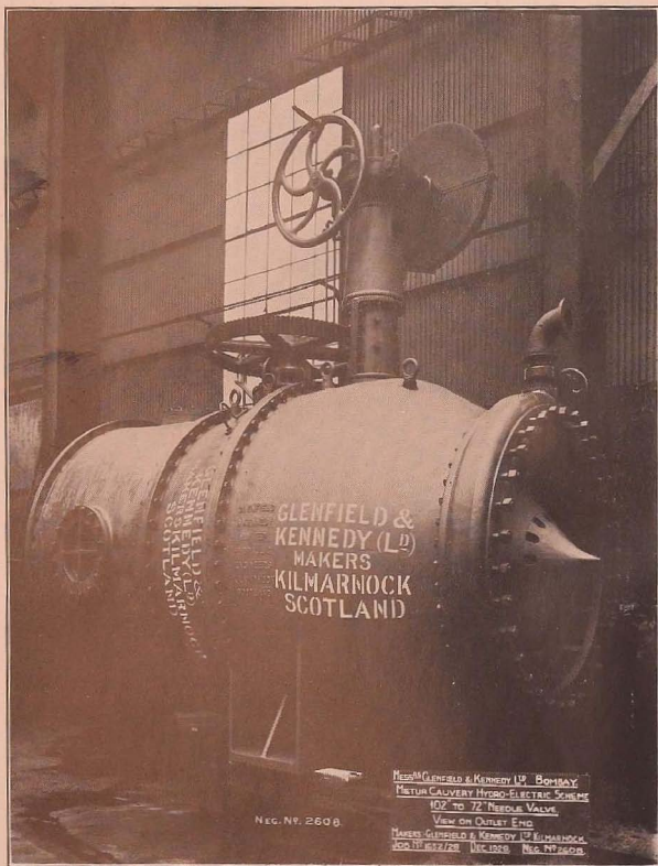
VIEW OF A NEEDLE VALVE.
