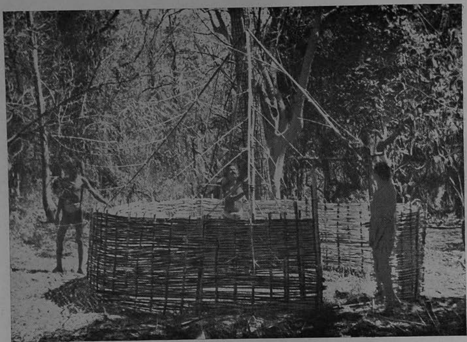
FIG. 42. Hitching the rafters over the forked centre pole.
