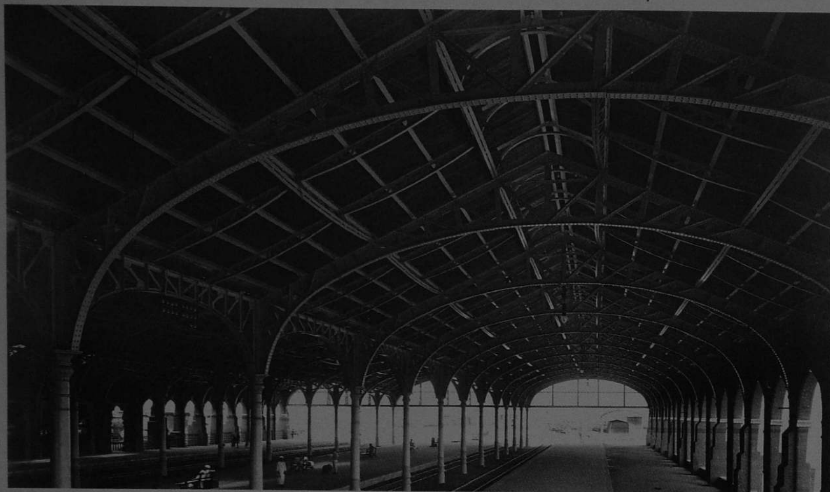
The platform looking east; Note the beautiful ironworks, the pillars were made by M/s John Lysaght Ltd., Bristol
