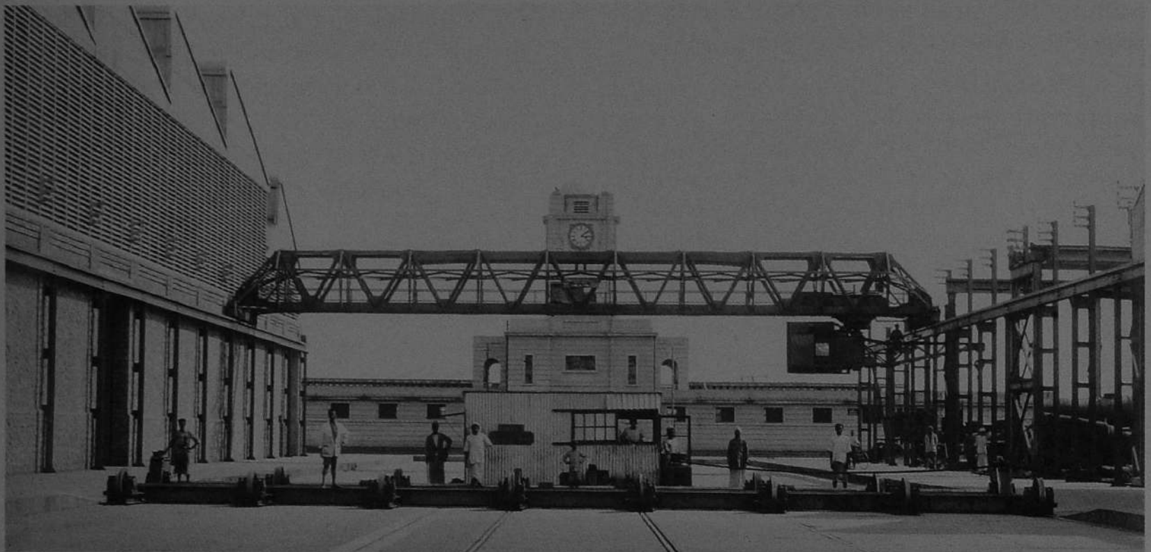
Traverser 'A' - showing 3 1/2 ton overhead electric travelling crane at Central Workshops, Golden Rock
