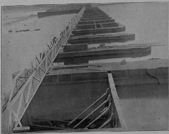
UNDER-SLUCICE GATES, SONE WEIR.
