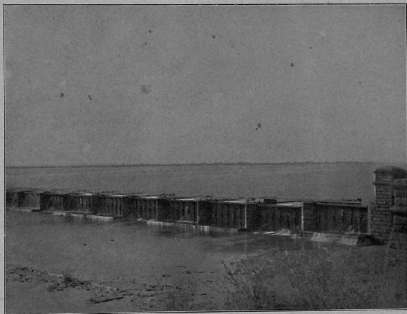
UNDER-SLUCICES OF THE SONE WEIR.
