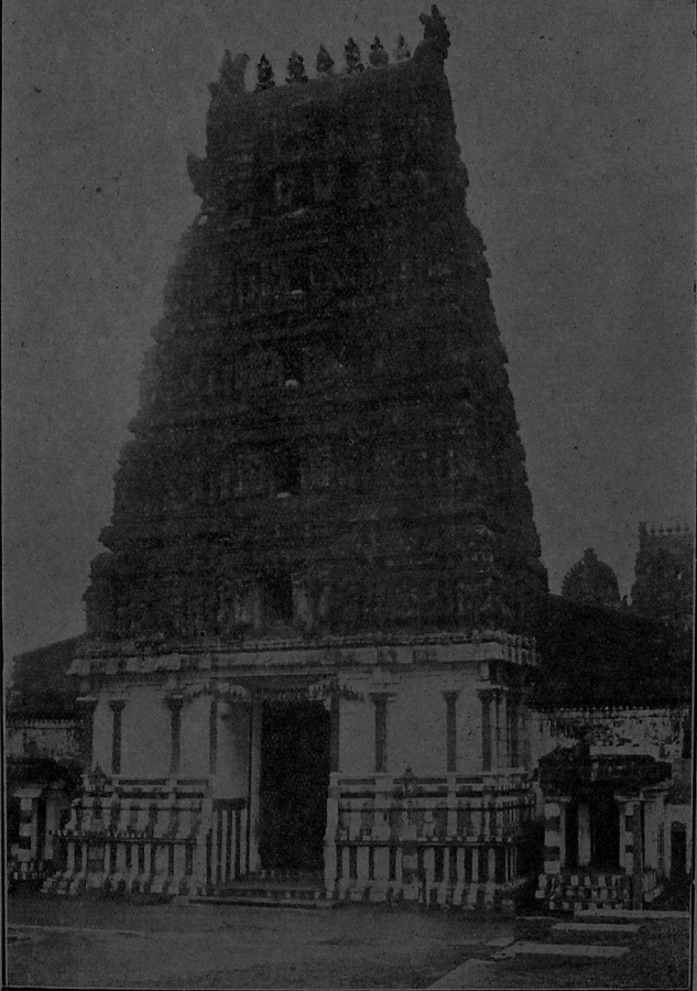
FIG. 10. THE SECOND EASTERN GOPURAM NAMED Rishi Gopuram
