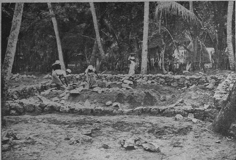
House construction in progress. The foundation is built of granite stones and random rubbles.
