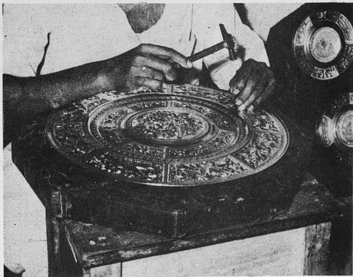
11. Art Plate fixed on a Wooden Plank before giving finishing touches.
